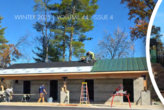
New restroom/showerhouse and playground at Charles Mill Lake Park Beach
