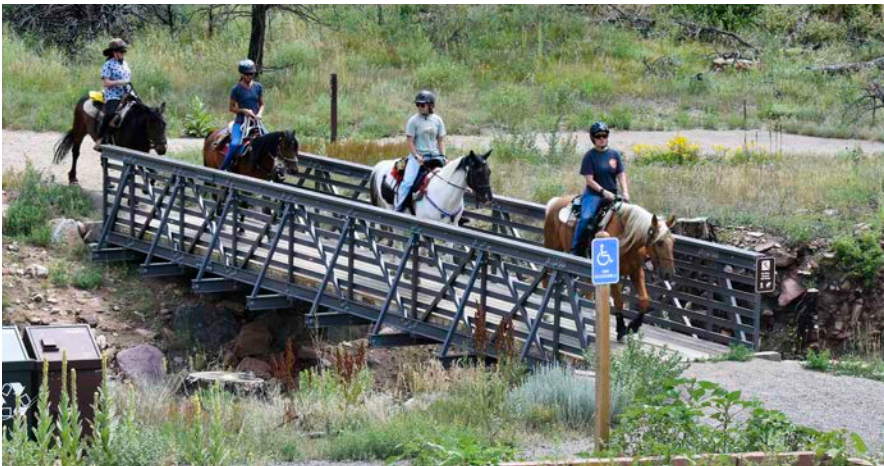
FRC bridges are very strong, fully capable trail bridges.
