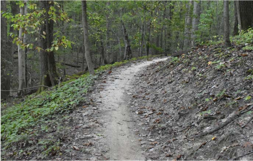
Good example—gentle backslope: A relatively recently built partial-bench biking-hiking trail with a gentle backslope resists sloughing, grows plants, holds fallen leaves and sticks, and blends into the site. (Also note that the fillslope revegetated.)
