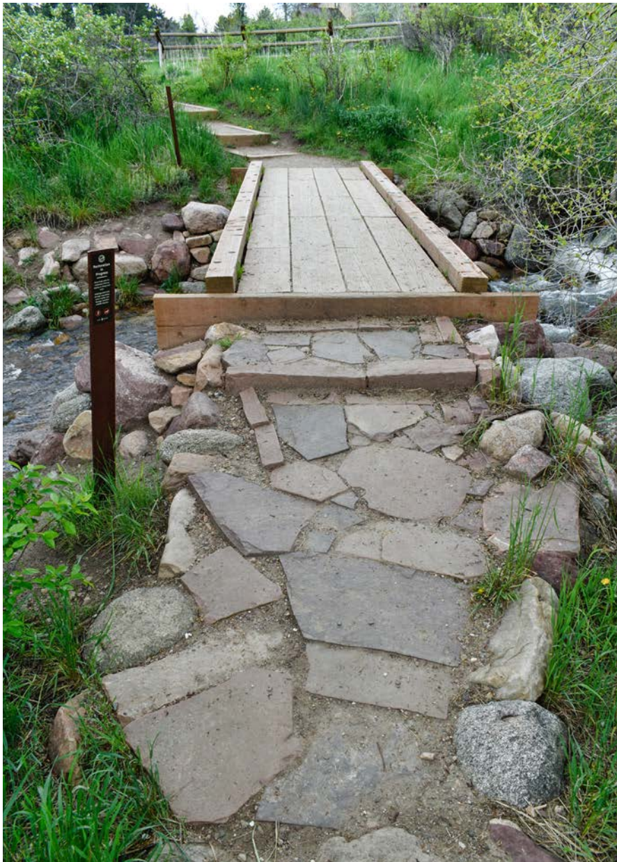
Ramp and bridge abutment seen from the side.
