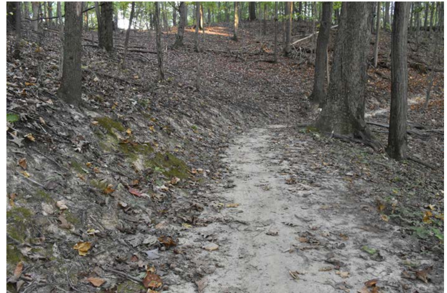
A partial-bench biking-hiking trail with a gentle backslope resists sloughing, grows plants and moss, holds fallen leaves and sticks, and blends into the site.
