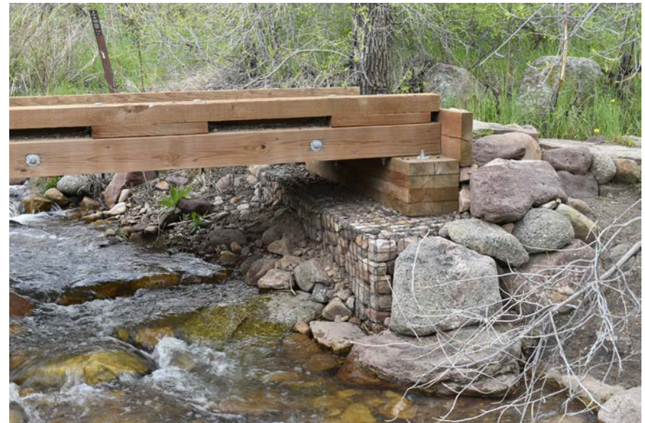
Ramp and bridge abutment seen from the side.
