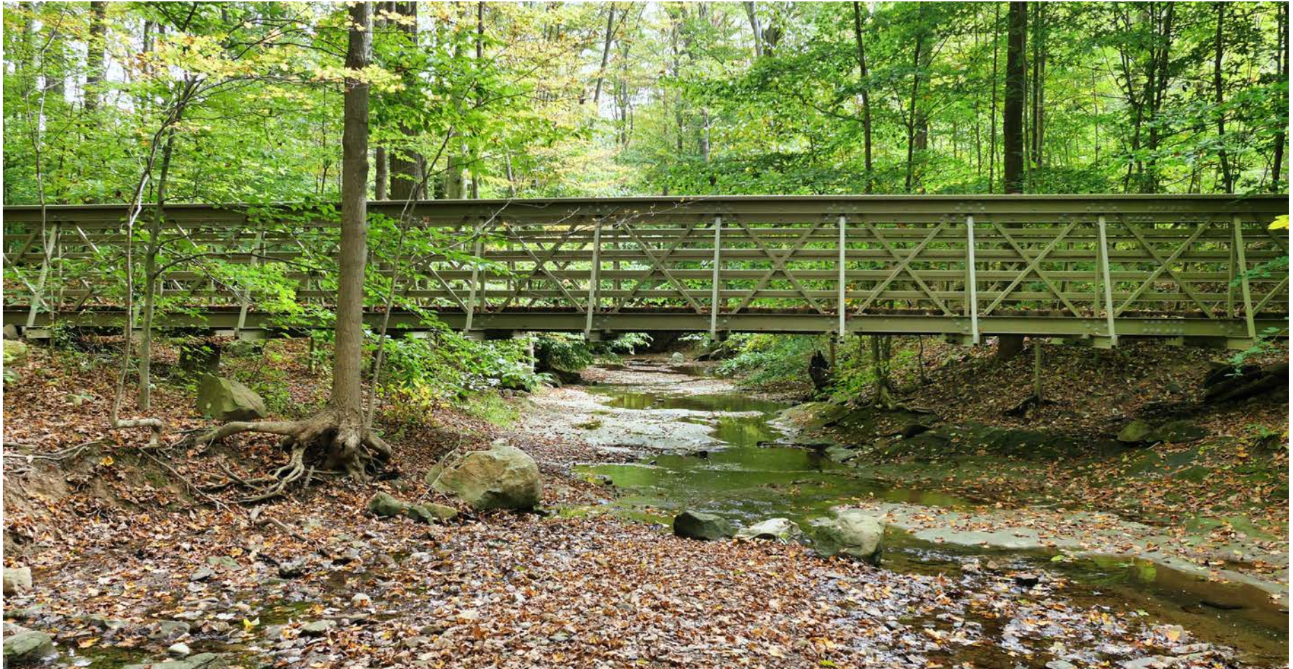
A 70-foot long, 4-foot wide FRC bridge on Buckeye Trail at Blue Hen Falls in Cuyahoga Valley National Park. The X-truss used in this bridge is the most attractive truss option
