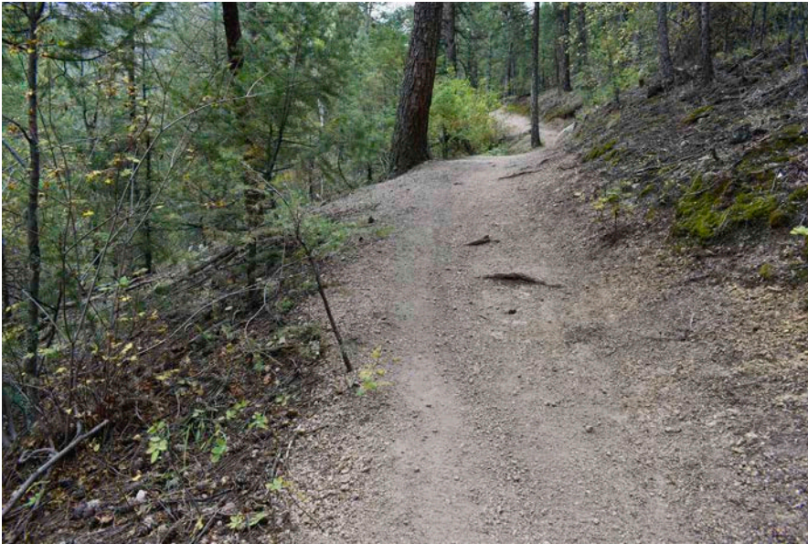
A partial-bench hiking-biking-equestrian trail with a rounded shoulder and creeping tread. Users avoid roots exposed by tread displacement by traveling on the outside edge, which creeps the tread onto the fillslope over time. Soil displaced from the tread lands on the shoulder, building up the shoulder as the tread sinks, enabling the entire tread to creep onto the shoulder over time.
