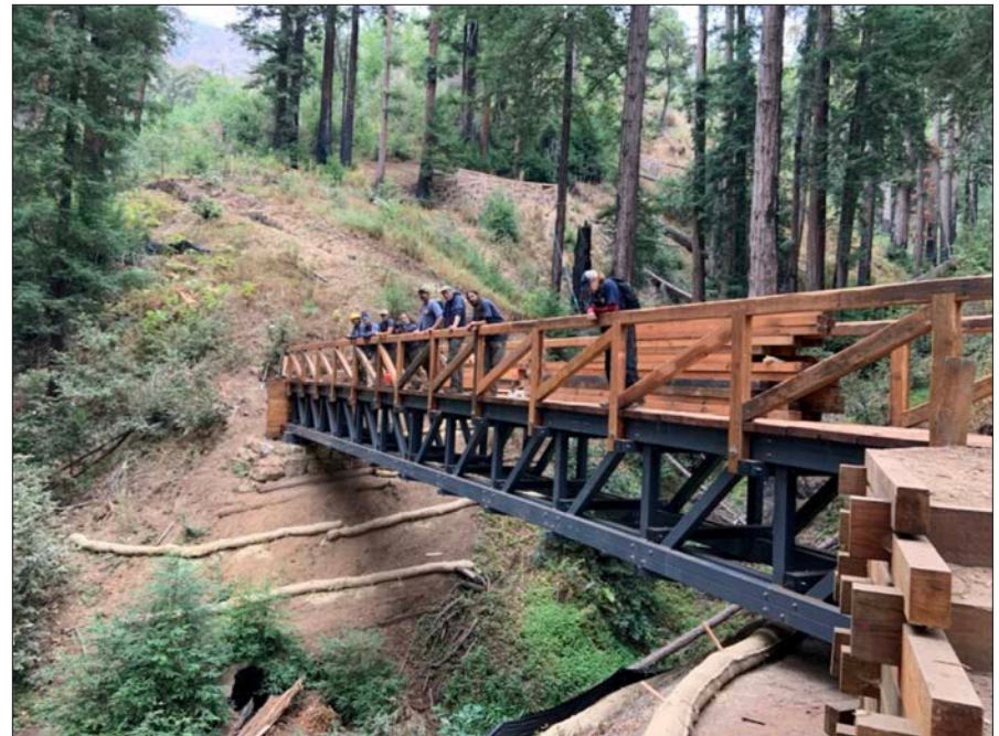
Two high bridges in Tappan and an 80-foot bridge in Pleasant Hill near Idlewood Cottage Area would be similar in form to this 70-foot fiberglass reinforced composite deck truss in Redwoods National Park. In a deck truss, the truss is below the deck and out of sight from users on the bridge. Railings would be a different style and the trusses would be a different color. (Photo by Wagners CFT US)
