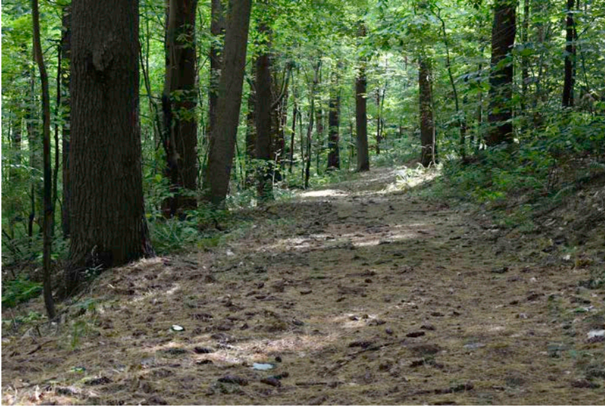
“Before”—Existing Hawk Ridge trail at Atwood is built like a small road. Its tread (travel surface) slopes downhill so much that it’s uncomfortable to walk on.
