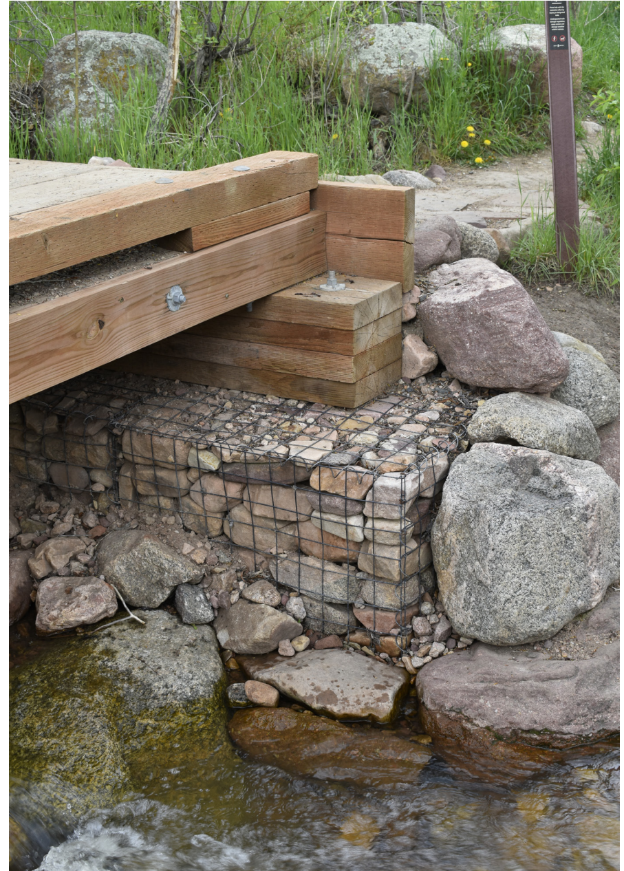
Bolt-laminated timber sills are bolted to zinc-plated gabions that are painted dark gray to minimize their appearance. The all-thread rod extending above the sill keeps the bridge from sliding off of the sills unless a flood lifts the bridge over the end of the rod. As of late 2025, this bridge has yet to be moved by a flood.
