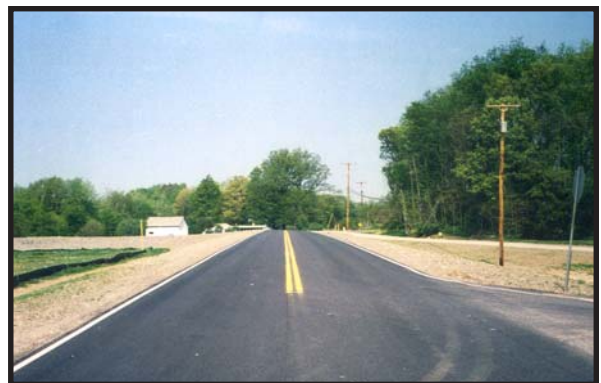
The MWCD will assist in projects that relocate or increase elevation for roads.
