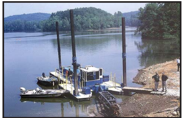
The dredge “Sedimental Journey” during its work at Charles Mill Lake.
