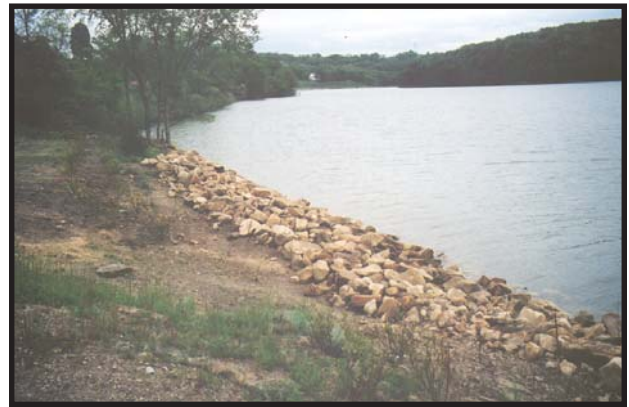
The MWCD will stabilize sections of the shoreline each year.
