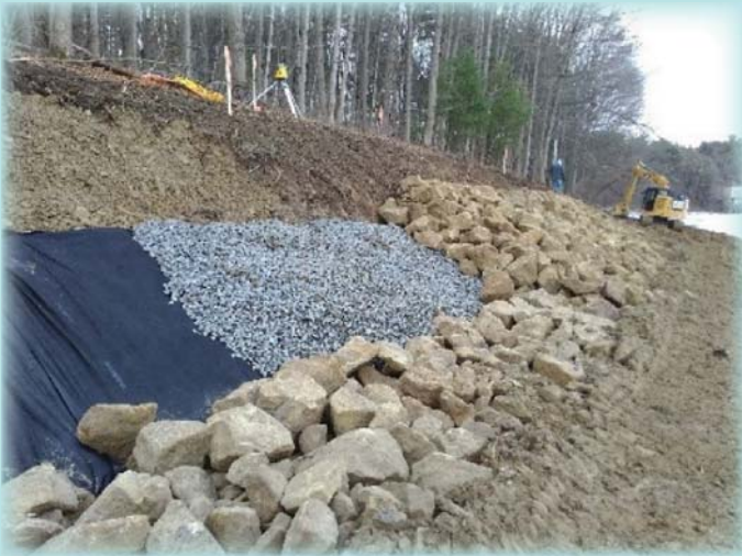
Tappan Highlands: Rock riprap with live stakes
