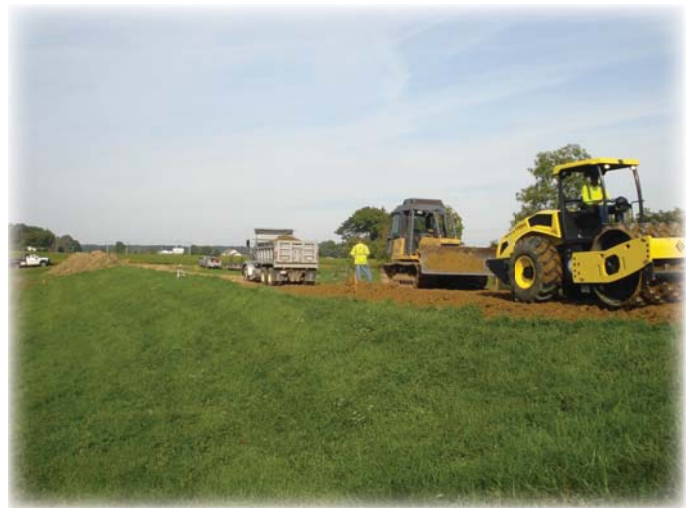
MWCD earthmoving crew raises the height of Chippewa Dam 5-D to meet new ODNR-Dam Safety requirements.
