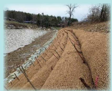
Seneca East Shore Cottage Area: Soil encapsulated lifts
