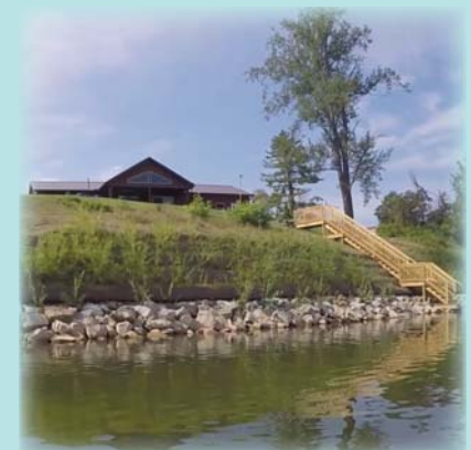
Seneca East Shore Cottage Area: Soil encapsulated lifts
