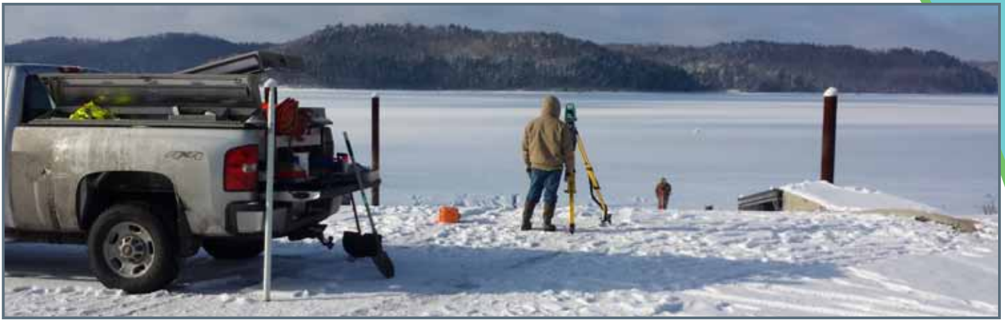
Base topographic and utility survey and mapping was completed by MWCD staff in the winter months in preparation of final design of capital improvement projects.
