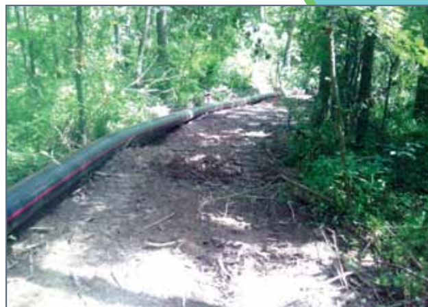
A temporary waterline at Seneca Lake depicts minimal land disturbance in conformance with the MWCD temporary water withdrawal agreement with Antero.
