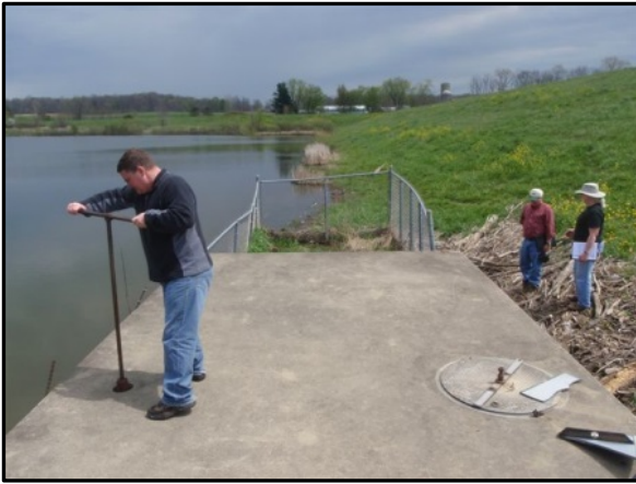
Bill Alderman, MWCD project accountant, opens a valve during the annual Chippewa dam inspection.
