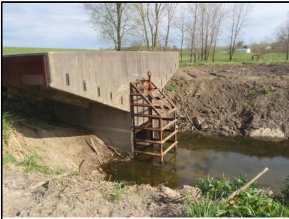
A new trash rack installed at Dam VIII-C.
