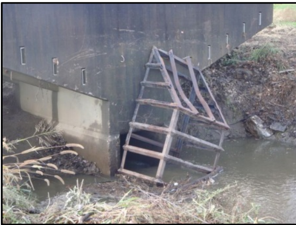
Failed trash rack at Dam VII-C.
