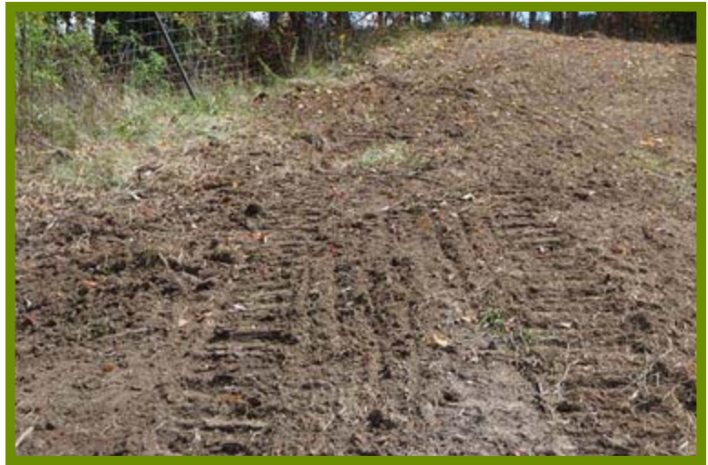
At Dam VIII-C, the eastern embankment of the dam was damaged by unauthorized All Terrain Vehicles or ATV's.
