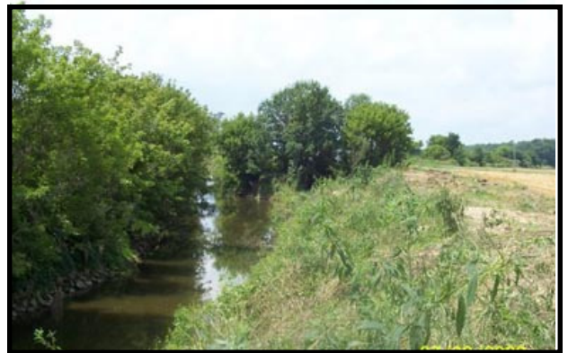
Trees and brush along the banks of Chippewa Creek between Shorle Rd. and Blough Rd. had grown over the years to the point where the flow of water was greatly reduced causing flooding of fields upstream.
