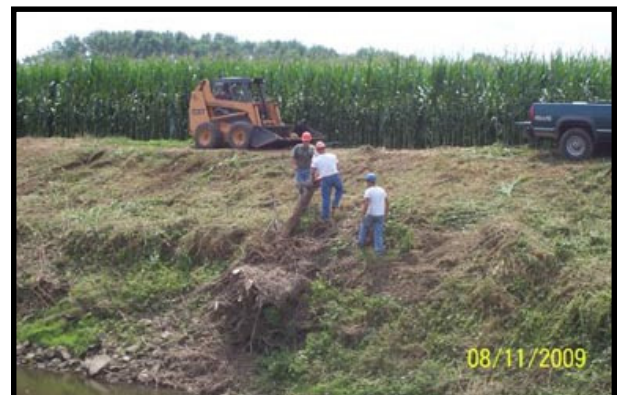
Photo above shows the crew clearing vegetation. In August of 2009, the trees and brush were removed along this section of channel. This area and all previously cleared sections will be mowed annually.
