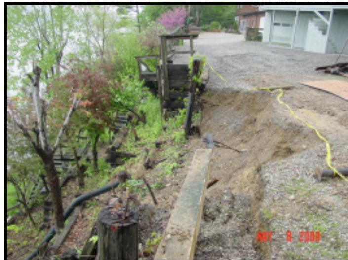
Severe erosion and slope stability concerns adjacent to residential structures at Pleasant Hill Lake in Ashland County have spurred a geotechnical investigation to determine the cause for slope instabilities. Thousands of tons of shoreline material have washed into Pleasant Hill Reservoir as a result of these instabilities.
