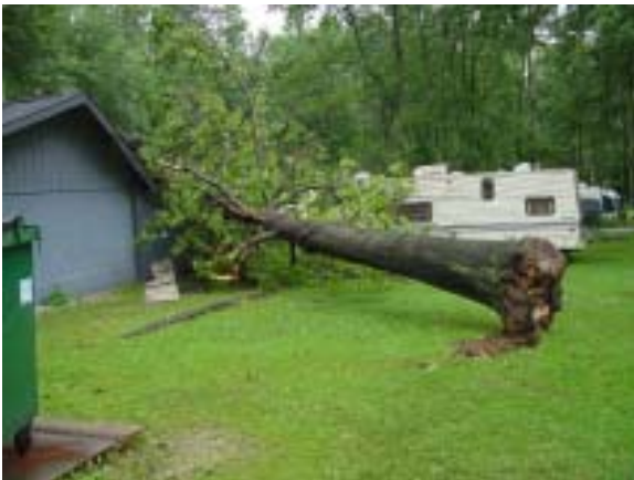
A shower building was among the damage sustained at Pleasant Hill Lake Park after a July thunderstorm.
