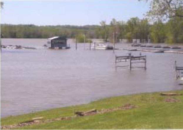
Spring rains in the Pleasant Hill Lake area left the marina at Pleasant Hill Lake Park inaccessible and closed the launch ramp for several days in mid-May.
