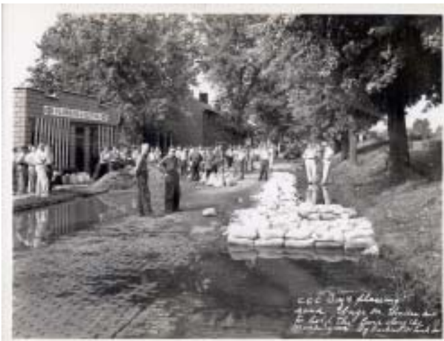
Neighborhood residents in the city of Zanesville receive assistance from the Civilian Conservation Corps in making and placing sandbags for protection from anticipated flooding in 1935.
