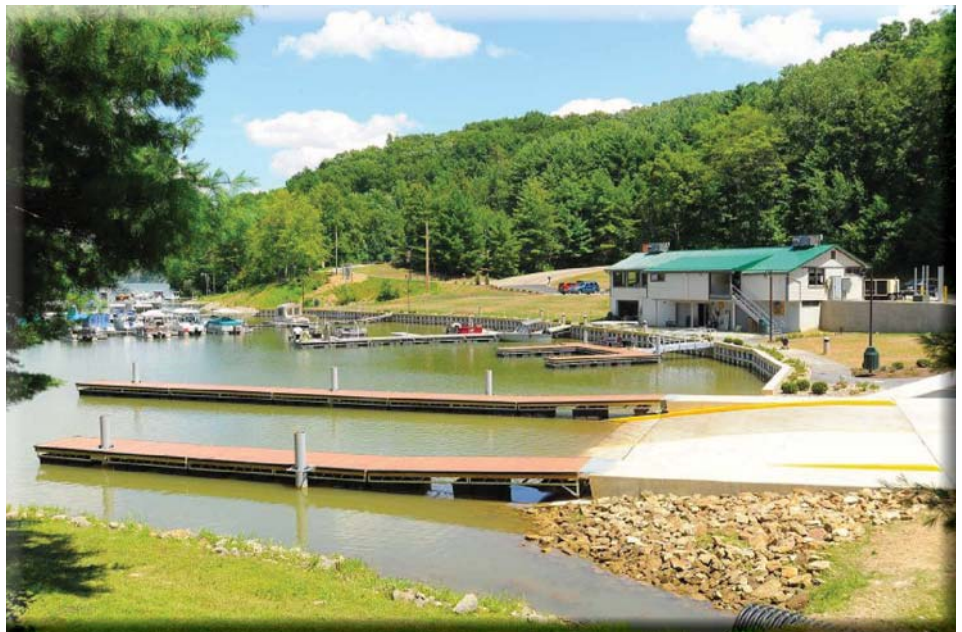
More than $1.6 million in renovations were made to Piedmont Marina this year, including a new boat launch ramp funded by the Ohio Department of Natural Resources Waterways Safety Fund.
