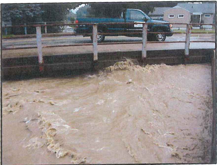
Figure 3: Looking south at East Sunset Drive bridge over Landis ditch, 2007
