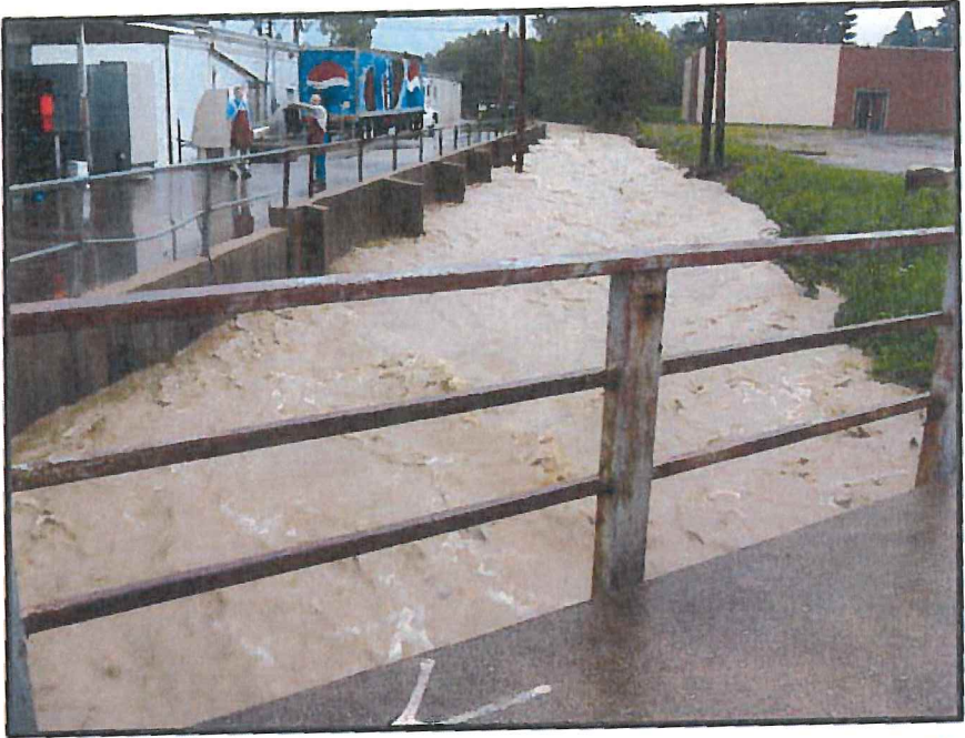
Figure 1: Looking north from the East Sunset Drive Bridge at flooding in Landis Ditch in 2007
