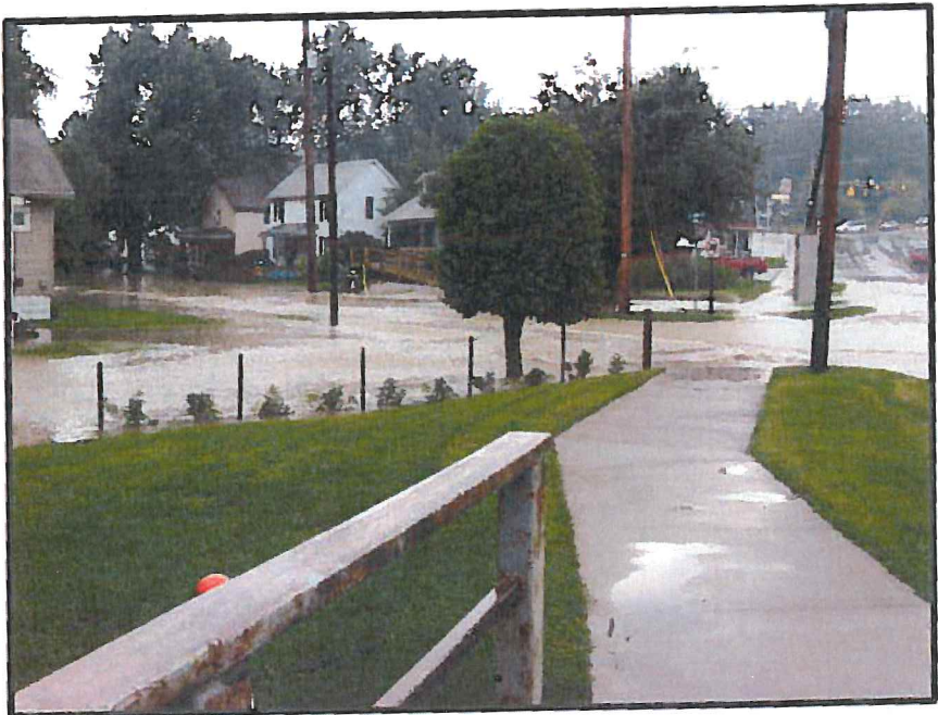
Figure 2: Looking west at flooding on North State Street and East Sunset Drive from East Sunset Bridge over Landis Ditch, 2007
