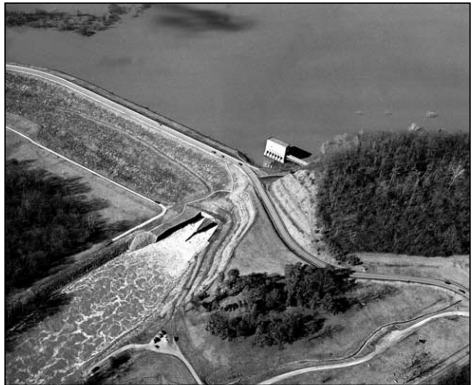
Mohawk Dam, located in Coshocton County just north of where the Walhonding River meets the Tuscarawas River to form the Muskingum River, is considered a priority for major rehabilitation by the U.S. Army Corps of Engineers.
