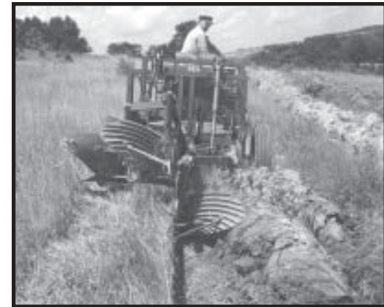
The rear view of the hydraulic-controlled 16-inch mold board double bottom two-way plow that was developed by H.P. Garritt, Soil Conservation Service forester with the MWCD. This view shows how the plow turns the contour ridges of small terraces preparatory to planting the trees. 1949
